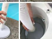
• Remove the basket from the skimmer and turn the red pointer of the main drain valve vertically. This will close the main drain and suction will be drawn solely from the skimmer.
